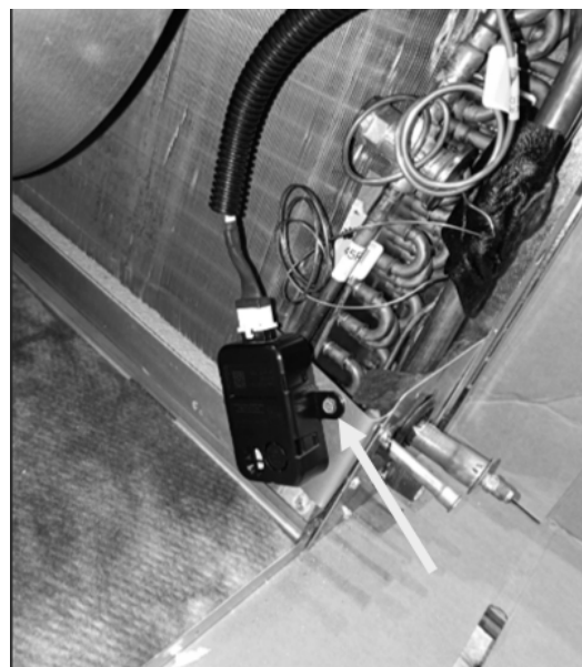
Figure 1 - Replacing Sensor to bracket
