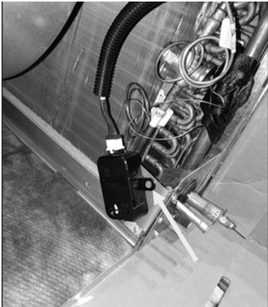
Figure 8 - Replacing Sensor to Bracket
